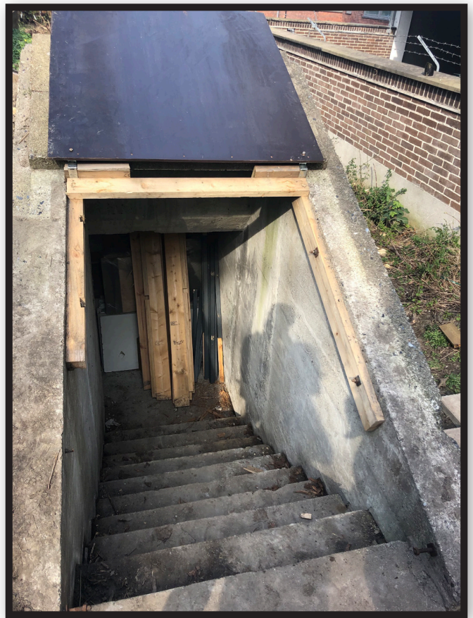
33: The entrance to one of the bunkers
